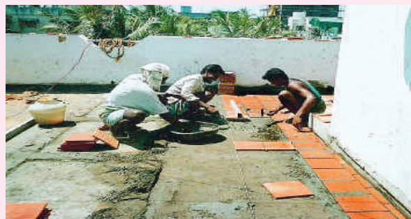
Mason fixing the tiles on the floor.
