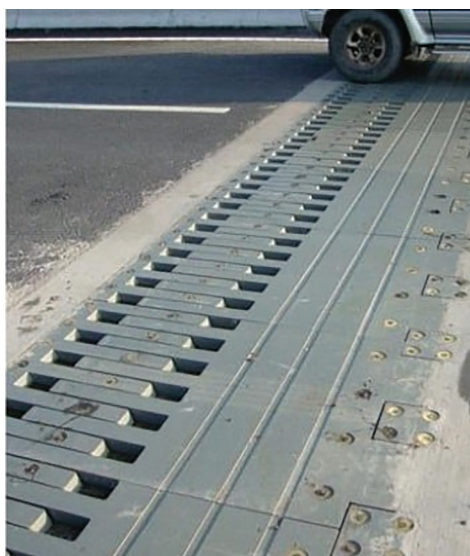
Figure 8.3 Expansion joints for safety
