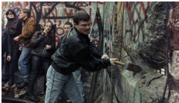
Demolition of Berlin wall
