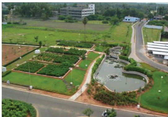
Fig .12.7 (a) DEWATS system at Auroville
